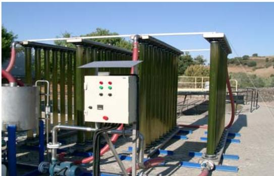
Fig.1: The first GreenAqua Prototype, based on LMMP technology.
